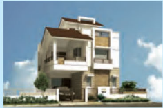
APARNA KANOPY LOTUS (Work in progress) 91 Value Villas, Gundlupochampally, Kompally
