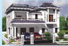
APARNA COUNTY (2008) 125 Independent villas, Hafteezpet
