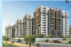
APARNA HILLPARK AVENUES (Work in progress) 647 Smart Apartments, Miyapur, Chandanagar
