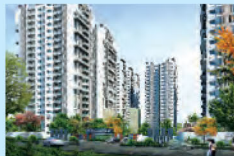
APARNA SAROVAR GRANDÉ (Work in progress) 720 Luxury Lifestyle Apartments, Nallagandla
