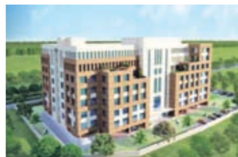
NIMAI TOWER Ready for Fit-Outs
