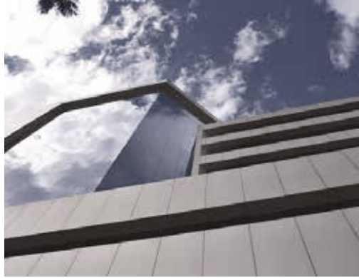
GODREJ CASTLEMAINE BUND GARDEN, PUNE
