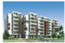
APARNA KANDOPY TULIP (Work in progress) 108 Wave apartments, Sundarapally, Madhapur
