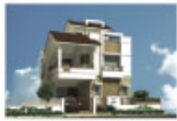
APARNA KANDOPY LOTUS (Work in progress) 91 Blue villas, Sundarapally, Madhapur
