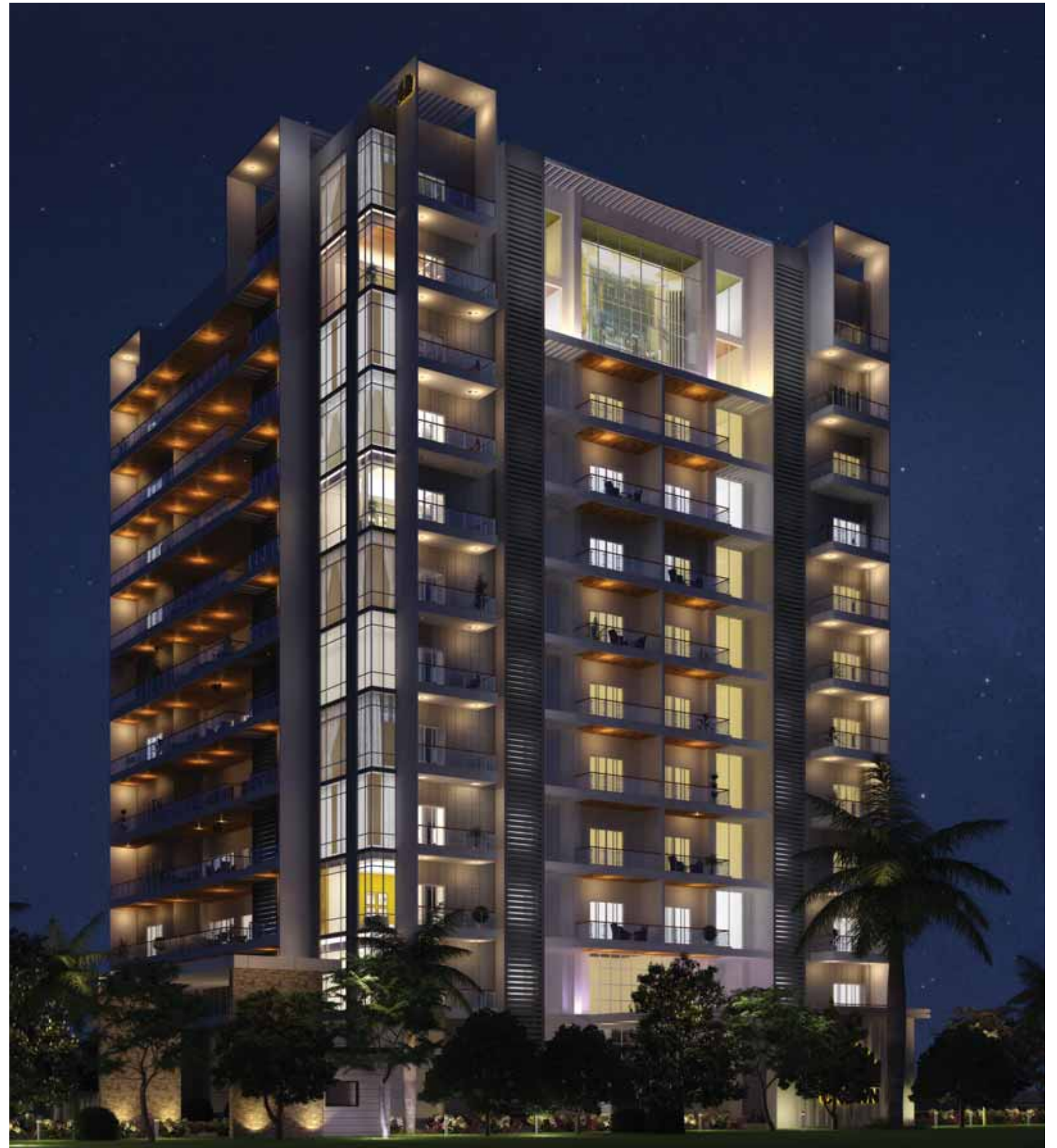
Top: Artist representation of night view of the building Plan approved and sanctioned by BBMP
