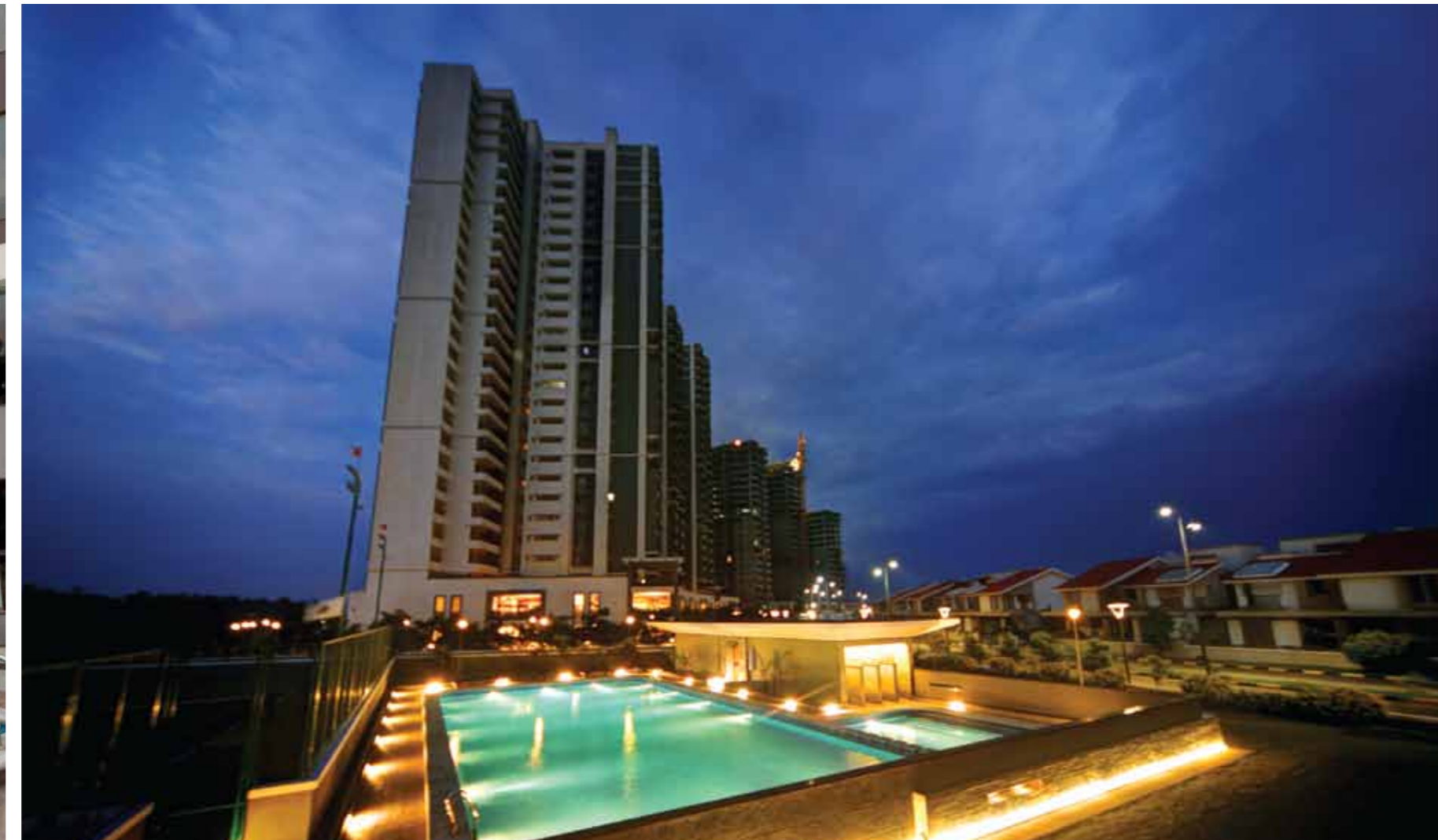
Sobha City, Thrissur, Kerala
