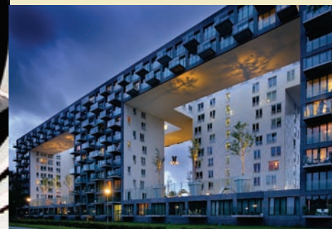
Parkrand Building, Amsterdam
