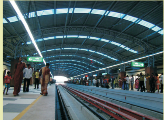
Kobi Najrul Metro Station
