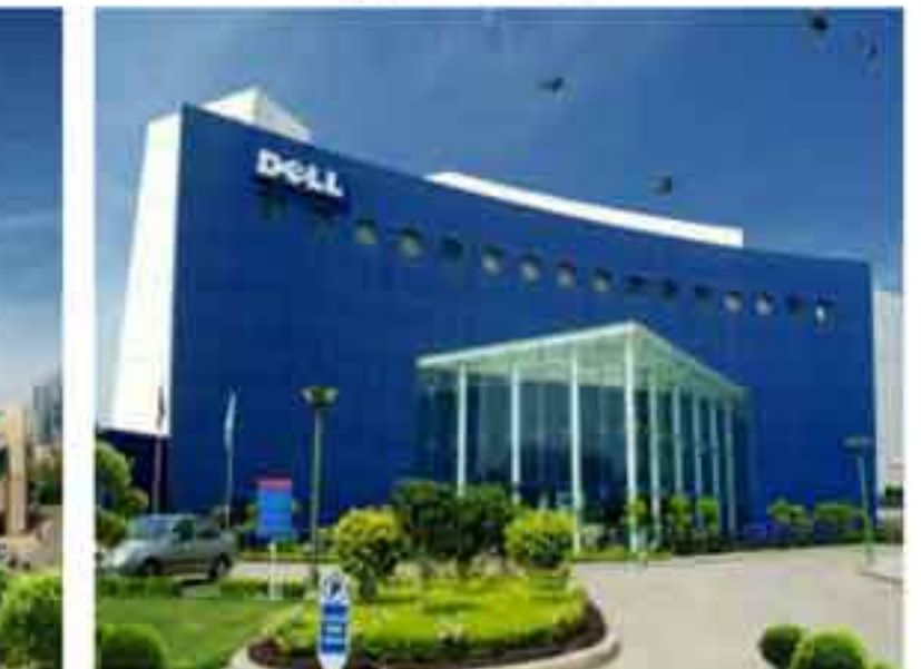
Vipul TechSquare, Gurgaon
