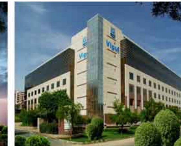
Vipul Plaza, Gurgaon
