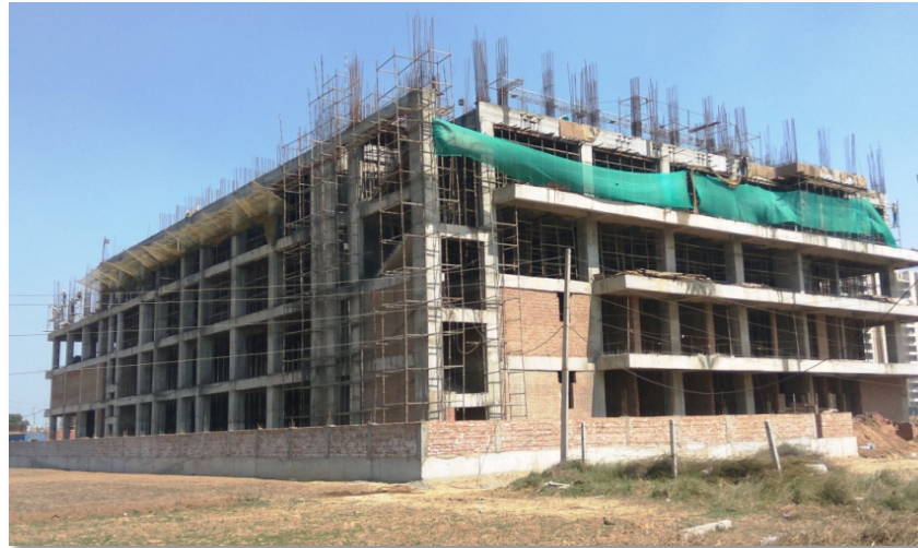
4 th Floor Roof Slab Casted
