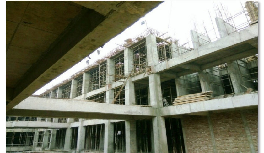
Atrium facing view
