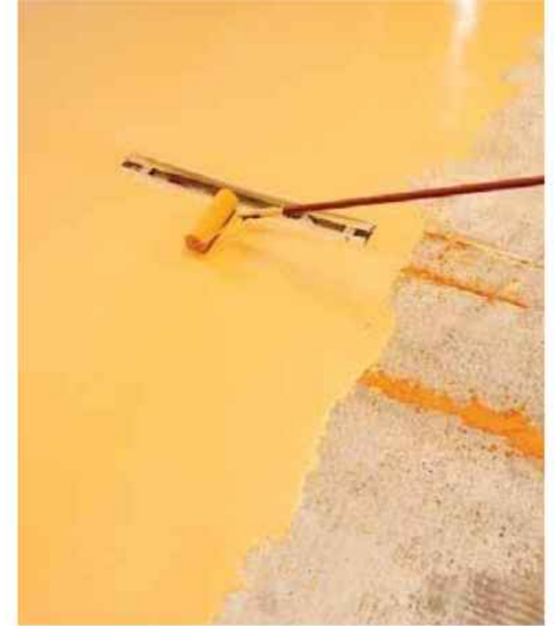
Waterproof coating up to 1.5 m in wet areas, more than 5 times of industry standard.
