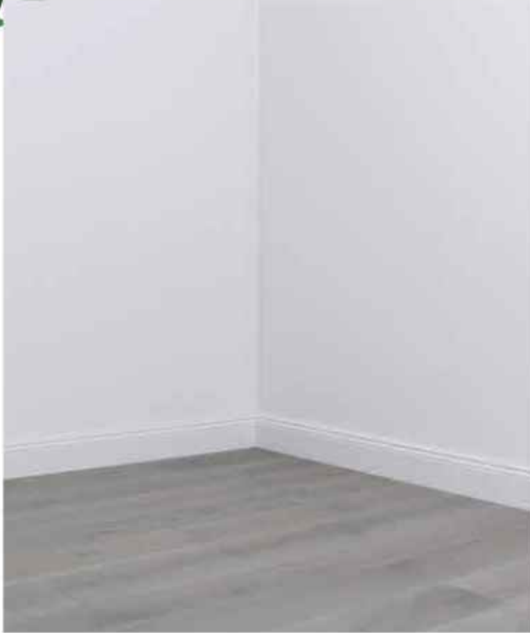
Application of anti-capillary coat on floor-wall junctions to prevent dampness
