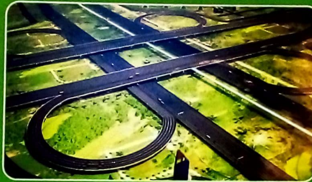
250 M WIDE 6 LANE AHMEDABAD-DHOLERA EXPRESS WAY
