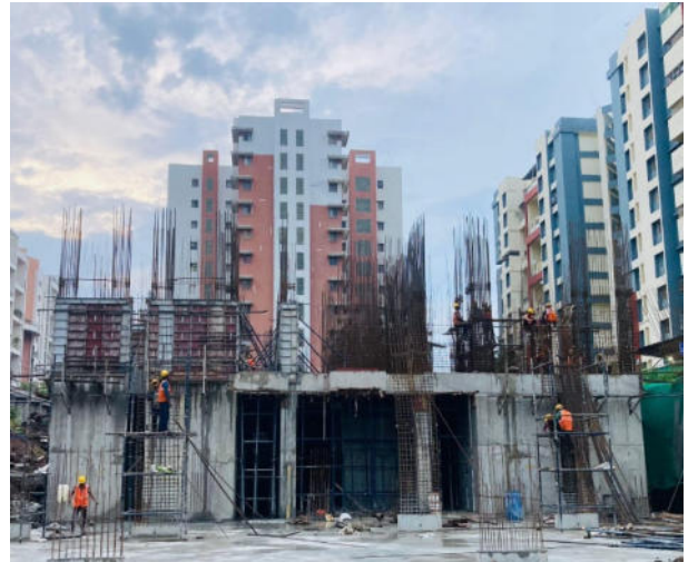
Figure 3: Portia Grande Tower 2 2nd slab wall Reinforcements completed and share wall casting in progress
