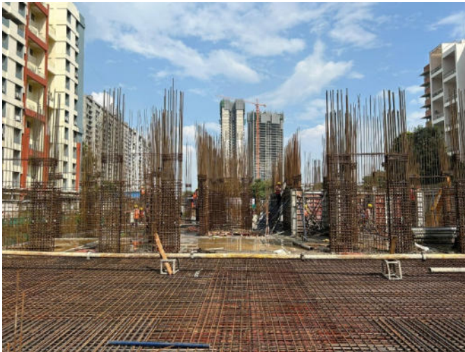
Figure 3: Portia Grande Tower 2 2nd slab wall Reinforcements completed and share wall casting in progress
