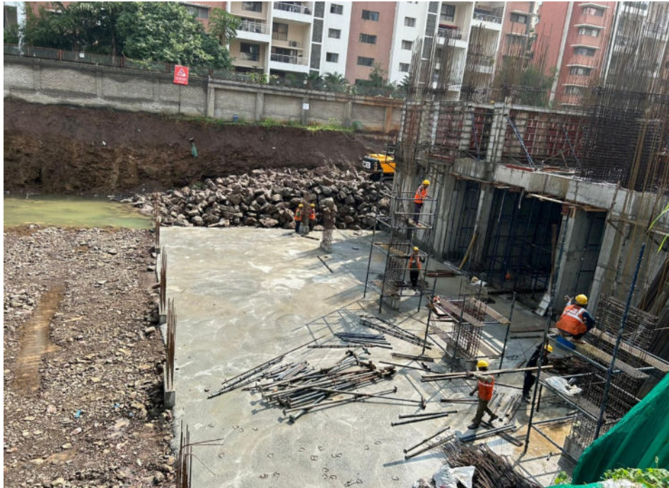
Figure 1: Portia Grande: Podium between T1 and T2 50% PCC completed and share wall reinforcement work in progress.
