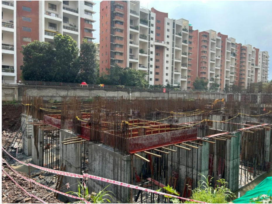
Figure 2: Portia Grande Tower 1 Ground floor slab shuttering work in progress
