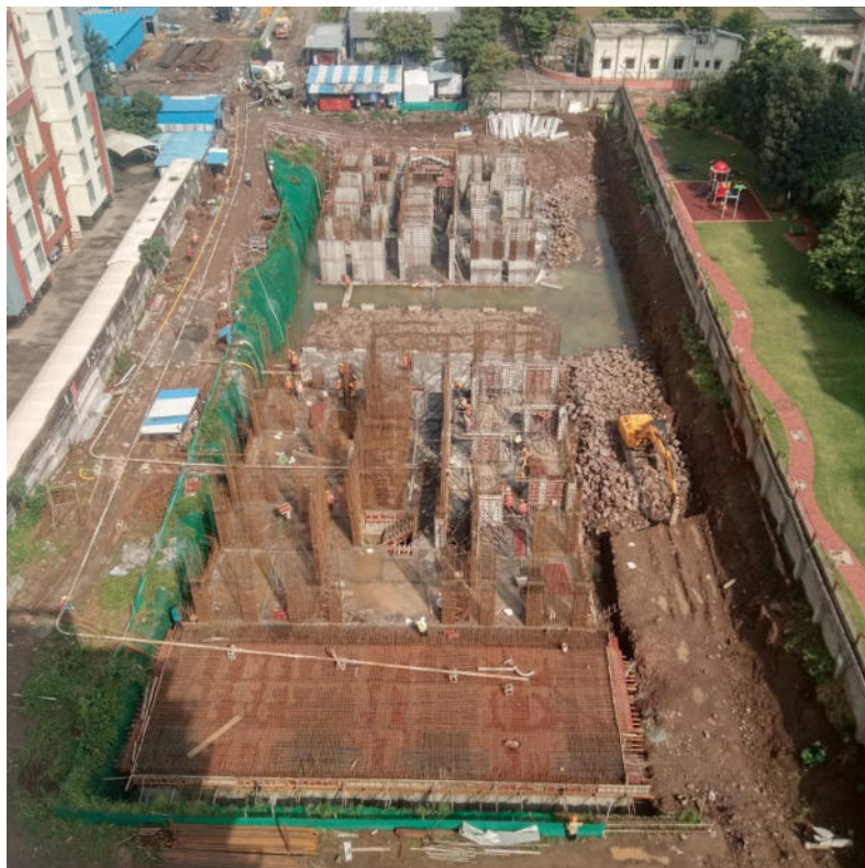
Figure 1: Portia Grande: Podium between T1 and T2 50% PCC completed and share wall reinforcement work in progress.
