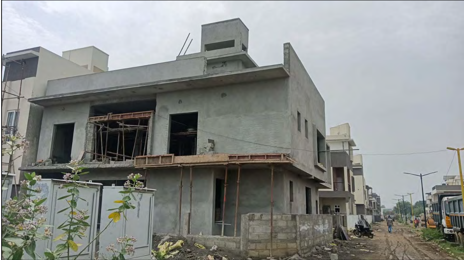
Villa 104 - Internal Plastering & External Plastering is on progress
