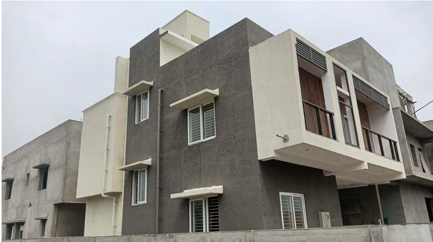
Villa 114 – 100% work completed
