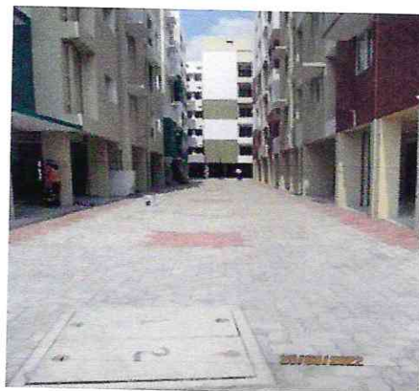
Paver Road work is completed COMPLETED
