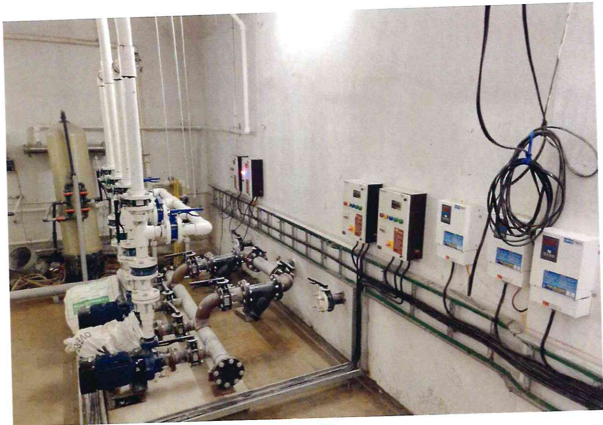
Water Treatment Plant (WTP)
