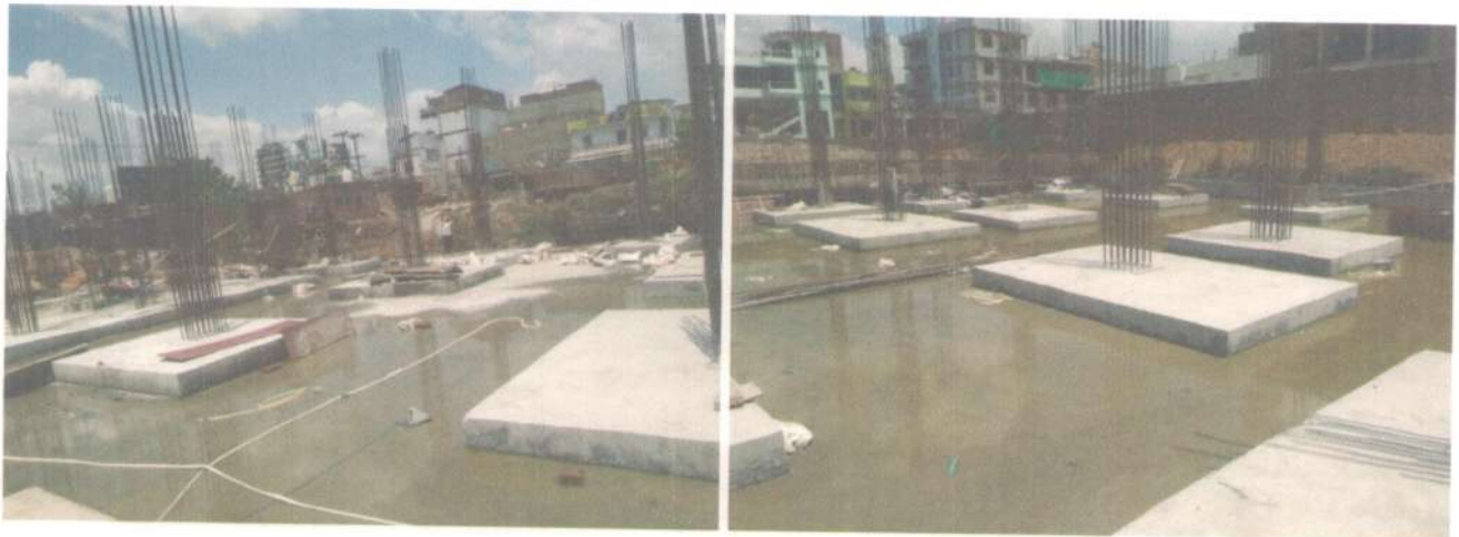
RAFT FOUNDATION CONCRETE WORK COMPELETE:-
