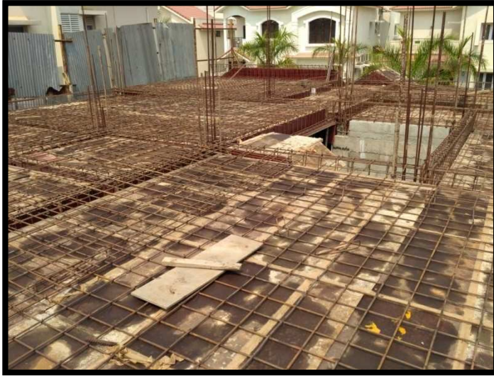
Villa# 581 Ground Floor roof slab rebar work completed.
