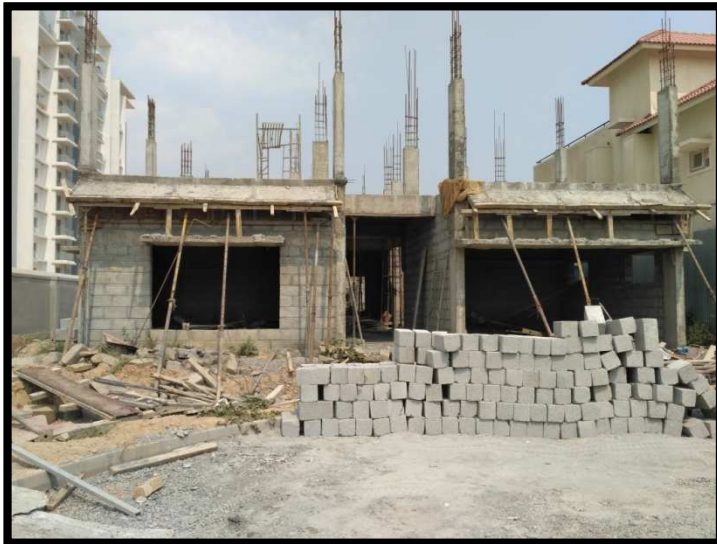
Villa# 638 First Floor Column concreting in progress.
