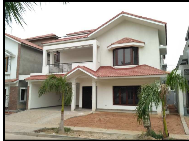
Villa# 784 Villa is ready for Final Hand Over
