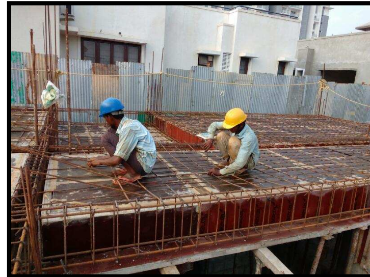
Villa# 642 GF rebar Work in Progress
