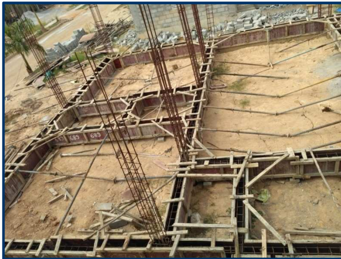
Villa# 695. Plinth Beam Shuttering in Progress
