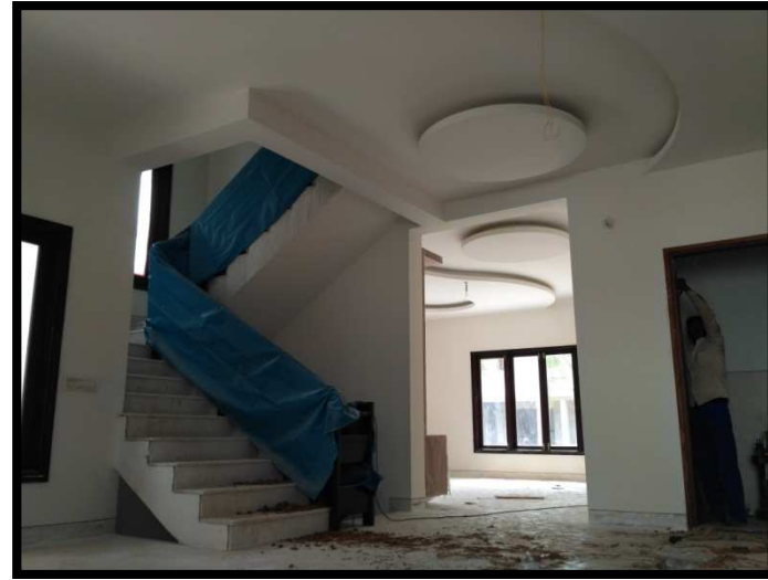
Villa # 664 Final finishing of walls after interior in Progress.
