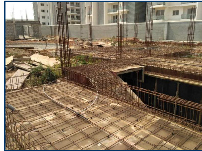
Villa # 662 Basement along with Plinth beam shuttering and rebar work in Progress.
