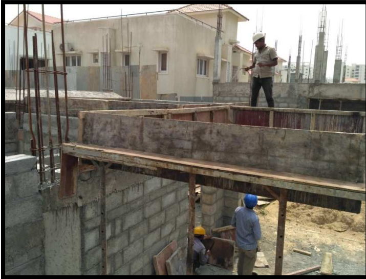
Villa# 661 Ground Floor Roof shuttering in progress
