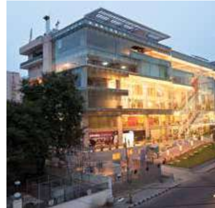
1 MG ROAD MALL Bengaluru
