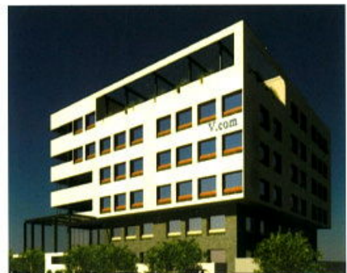
IT space Commercial Building, Electronics City
